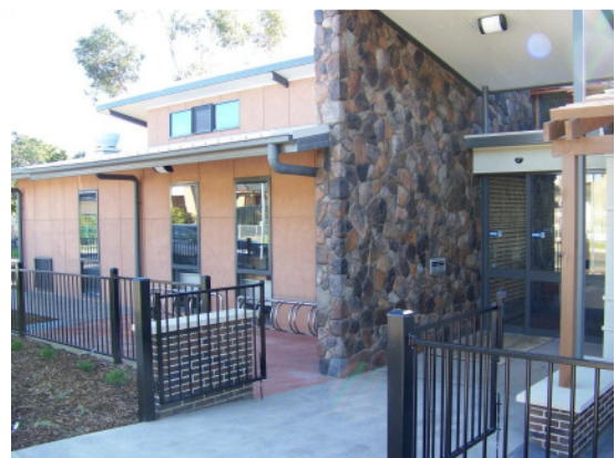
The carbon neutral East Reservoir Neighbourhood House
