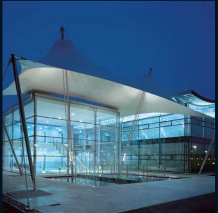
THE DYSON RESEARCH, DESIGN AND DEVELOPMENT FACILITY IN WILTSHIRE, UK.
